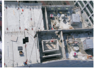
Figure 25. Erection of solid slab with welded plates
