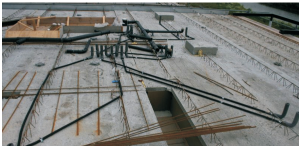
Figure 40. Plumbing pipes in topping of plank floor
