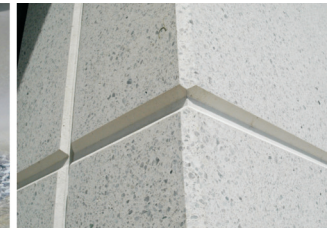
Figure 8. False joints in precast panel
