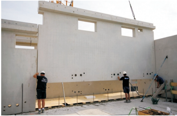
Figure 37. Several openings in precast wall panel
