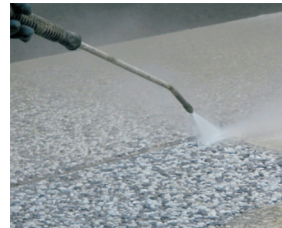
Figure 7. Exposed aggregate finish
