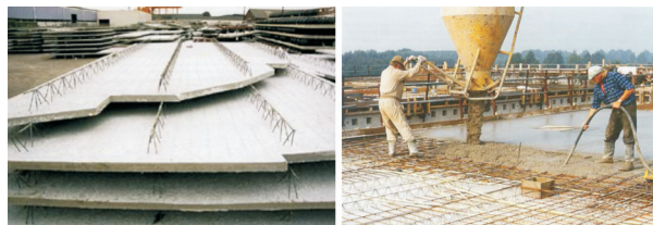
Figure 22. Various precast slab shapes Figure 23. Casting of concrete topping
