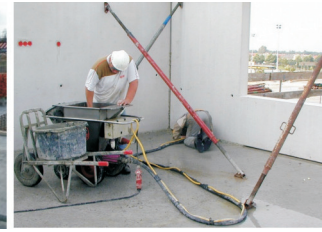
Figure 33. Pumping grout in horizontal joint
