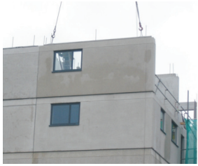
Figure 3. Large precast exterior wall panels
