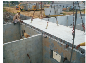
Figure 26. Solid slab with protruding reinforcement
