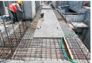
Figure 27. Solid slab with stitching reinforcement
