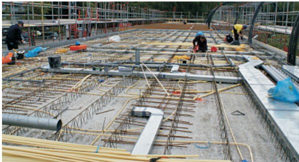
Figure 39. MEP services in topping of plank floor
