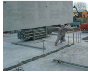
Figure 32. Placing wall in mortar bed
