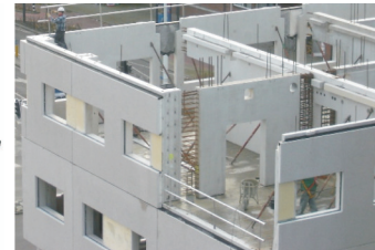
Figure 35. Vertical connections between internal walls
