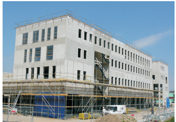
Figure 2. Large precast panel construction
