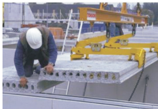
Figure 11. Hollow core slabs
