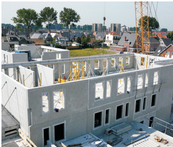
Figure 1. Large precast panel construction
