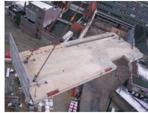
Figure 24. Solid slab with welded plates
