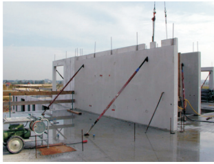
Figure 4. Large precast interior wall panels
