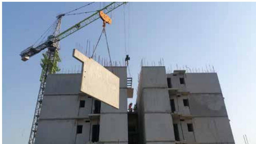
(Picture 2. Precast concrete wall erection)
