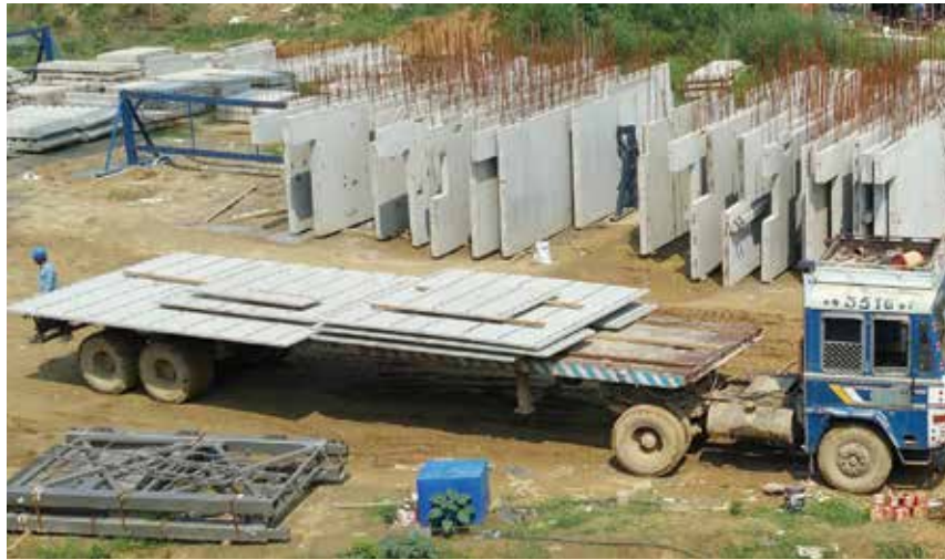
(Picture 16. Transport of precast slabs)
