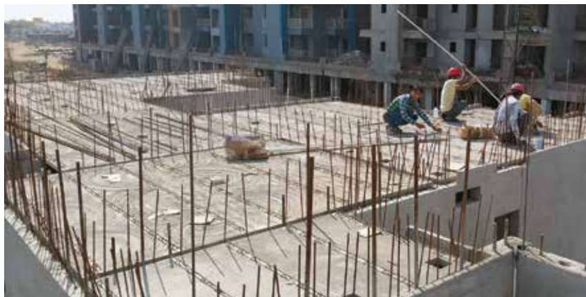
(Picture 4. Precast half slabs with lattice girders)
