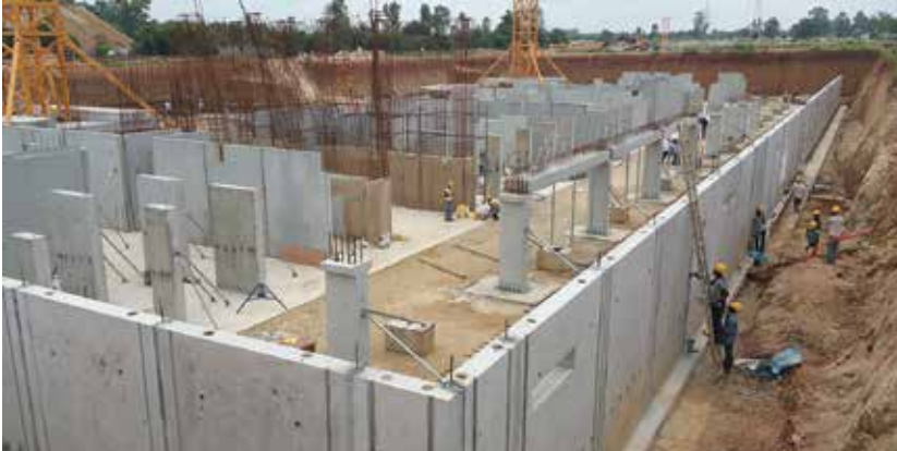
(Picture 22. Basement structure with precast retaining walls)
