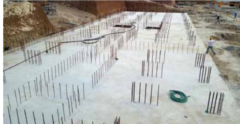
(Picture 18. Foundation raft with starter bars for precast columns and walls)
