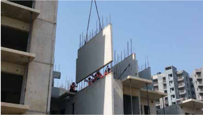
(Picture 6. Erection of load bearing precast wall panel)
