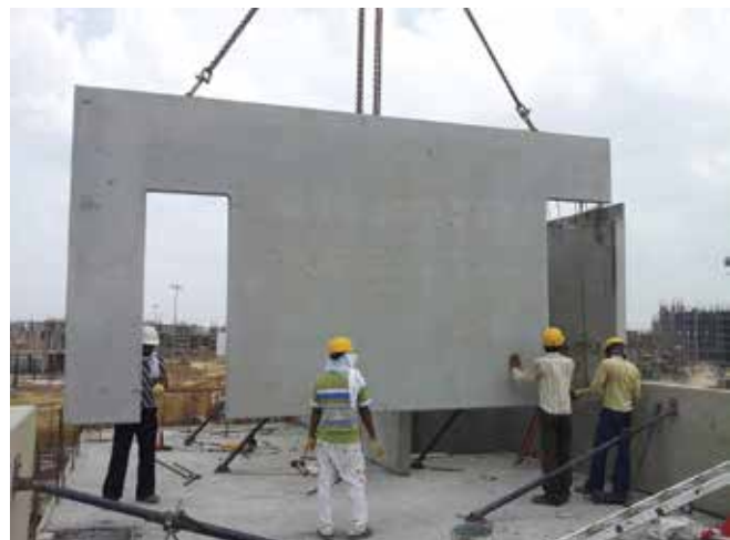
(Picture 33. Erection of precast partition wall panel)
