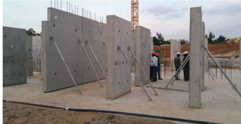
(Picture 19. Basement precast walls and columns)
