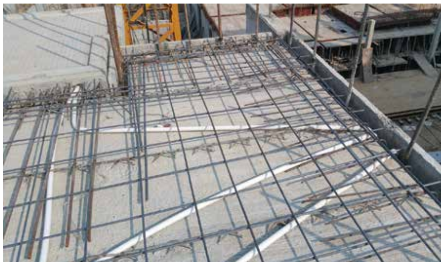
(Picture 7. Half slab top reinforcement lapped with protruding wall and balcony reinforcement)
