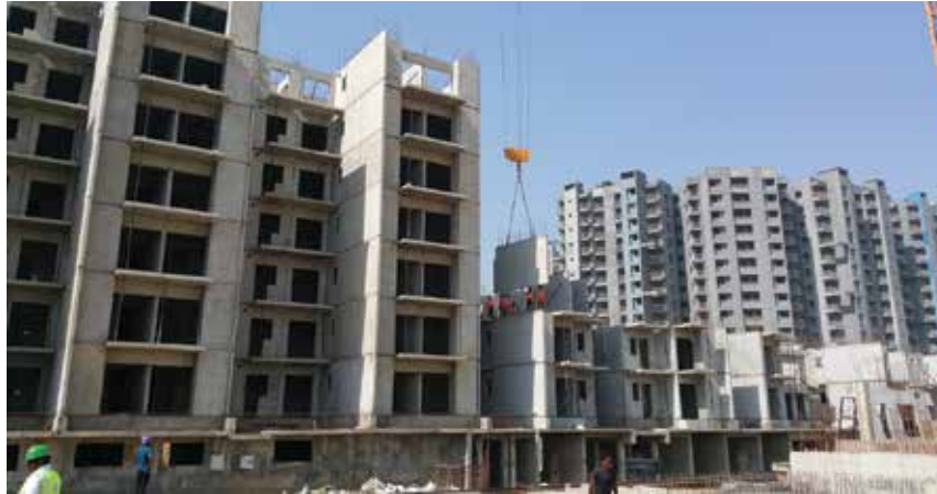
(Picture 3. Precast concrete load bearing structure on top of basement)
