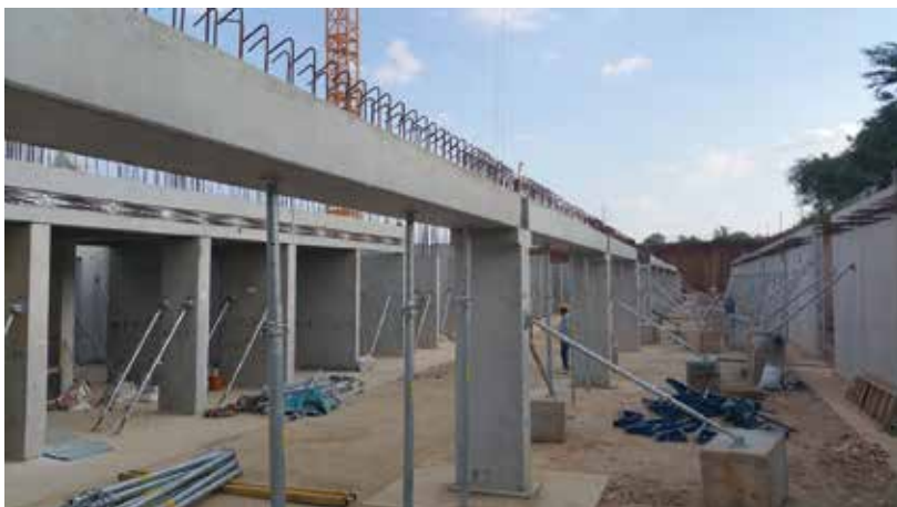
(Picture 20. Extended basement structure with precast columns and half beams)
