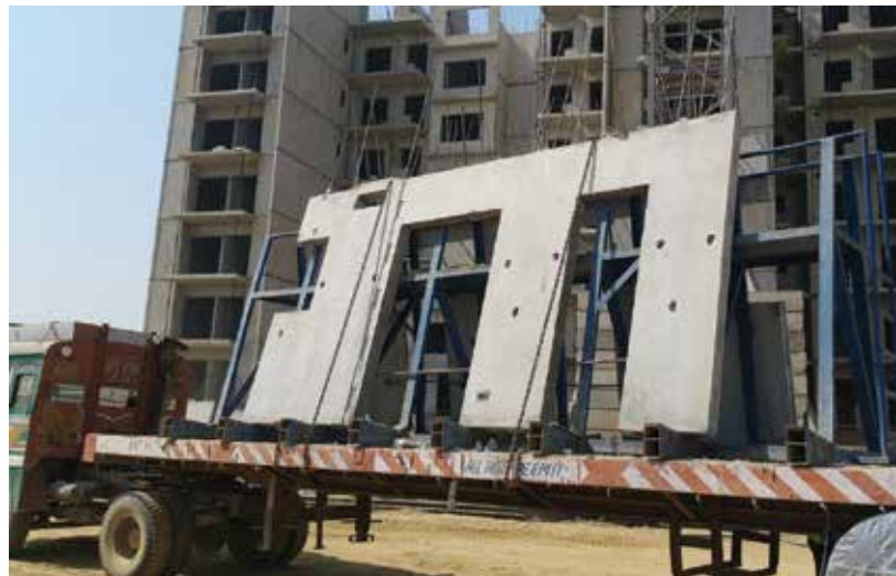
(Picture 15. Transport of precast wall panels)
