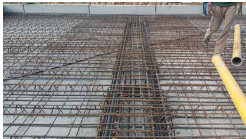
(Picture 21. Extended basement structure with precast half beams and half slabs)
