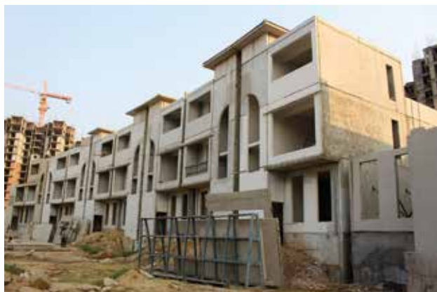
(Picture 36. Villas constructed with large precast panels)
