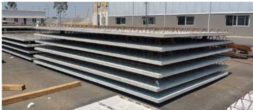
(Picture 30. Stacking of half slabs)
