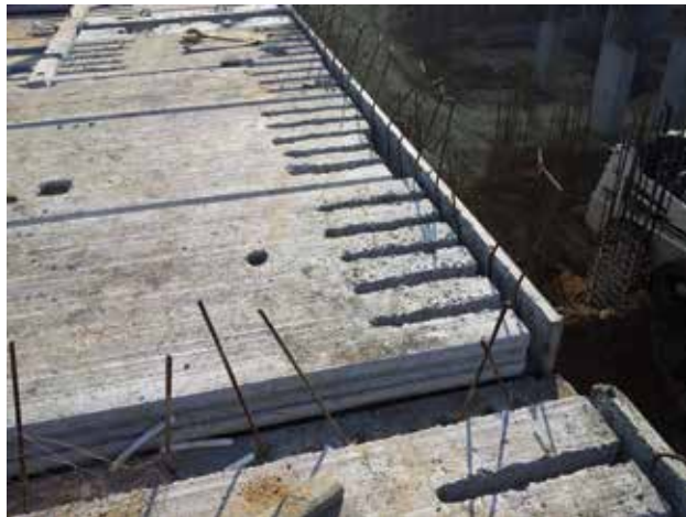
(Picture 34. Precast hollow core slabs with connection to precast walls)
